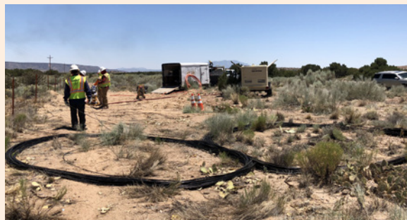
Fiber crews coil the fiber optic cable in large figure eights in preparation to blow the fiber between pull boxes located approximately 2000' feet apart. The process is repeated every 1-2 pull boxes for the 30-mile route.
